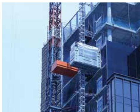
management and diagnosis, a lateral door option and being able to configure the hoist. A new square mast - the M650 - has been designed which has the capacity for two hoists, doubling the load capacity and allowing operators to work on different floors.
