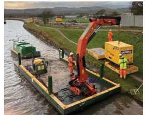
waterway bed. This set-up is similar to ocean going 'jack up vessels', in which the jacks can lift the boat out of the water but is only possible at pre-set inboard spacings. Outrigger type legs excel in providing a wide footprint for good lateral stability. However, unlike their vertical counterparts, they cannot be used to lift boats out of the water."
